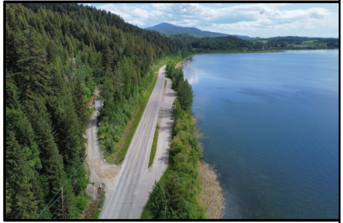
Access May 30 th 2023: Drone View of Existing Boat Access Area
