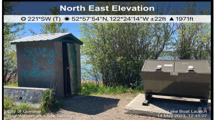
Access May 14 th 2023: Existing Outhouse Structure
