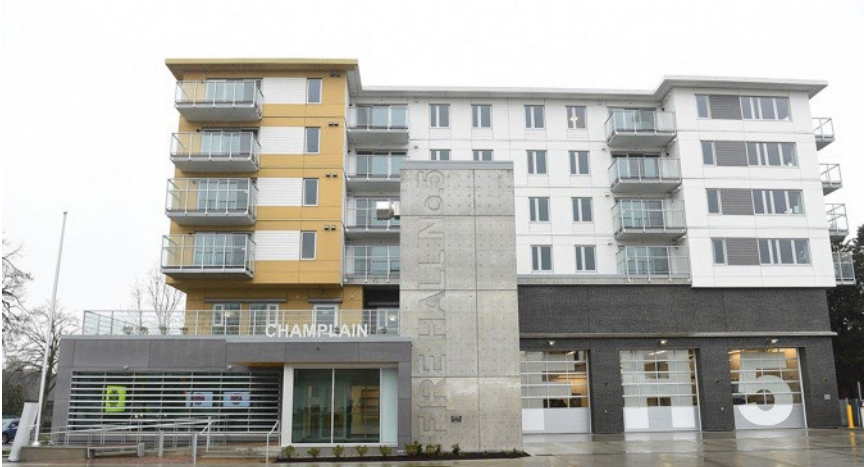
Vancouver Fire Hall #5 & Social Housing
