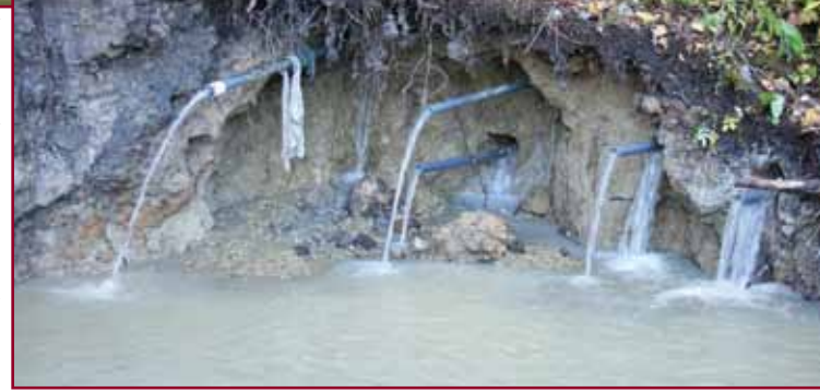
The first phase of the West Quesnel Land Stability Dewatering Program has been installed. Crews were active throughout 2012 drilling vertical pumping wells (above) and drains, and installing storm water upgrades. At right is a photo of a few of the more than 70 horizontal drains shortly after they were drilled. The water is collected and taken out of the Land Stability study area.
