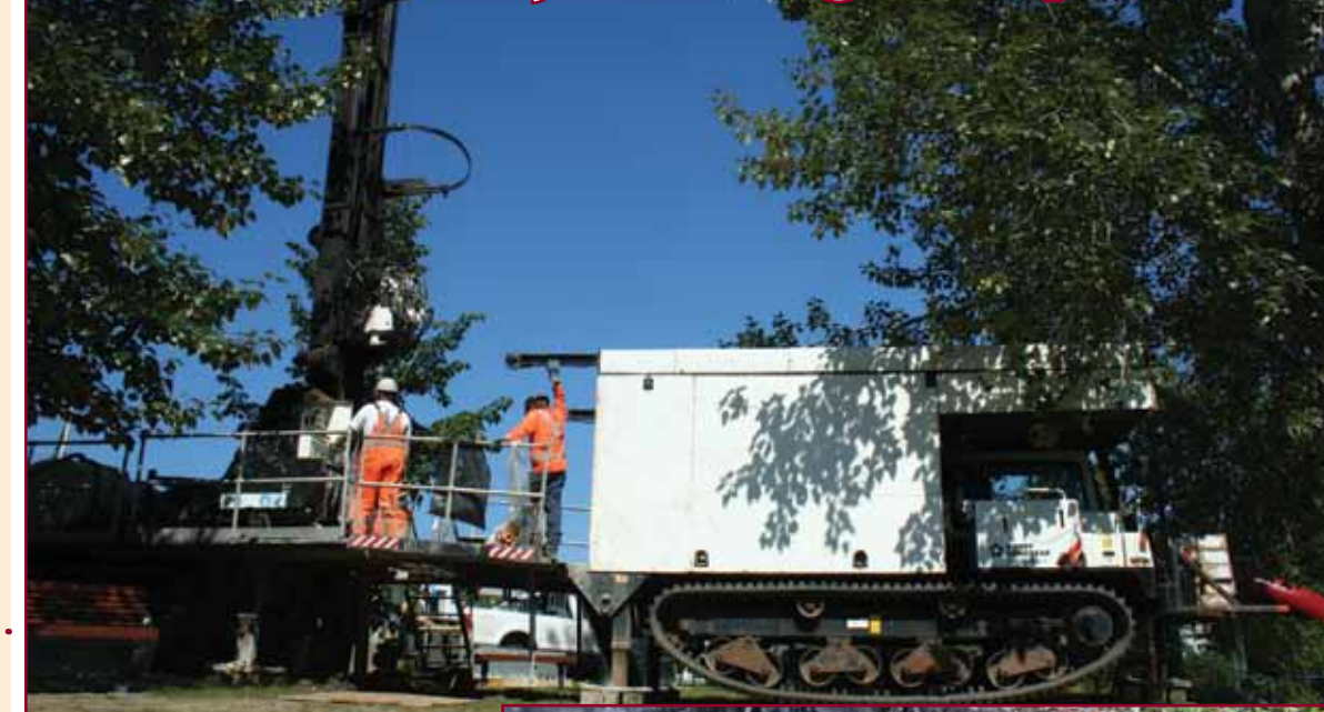
The first phase of the West Quesnel Land Stability Dewatering Program has been installed. Crews were active throughout 2012 drilling vertical pumping wells (above) and drains, and installing storm water upgrades. At right is a photo of a few of the more than 70 horizontal drains shortly after they were drilled. The water is collected and taken out of the Land Stability study area.
