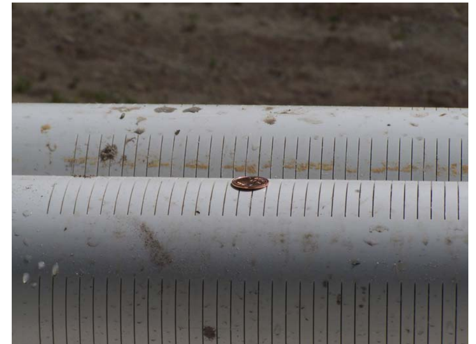
Photo 6: Well screen installed at PW4 and PW5.
