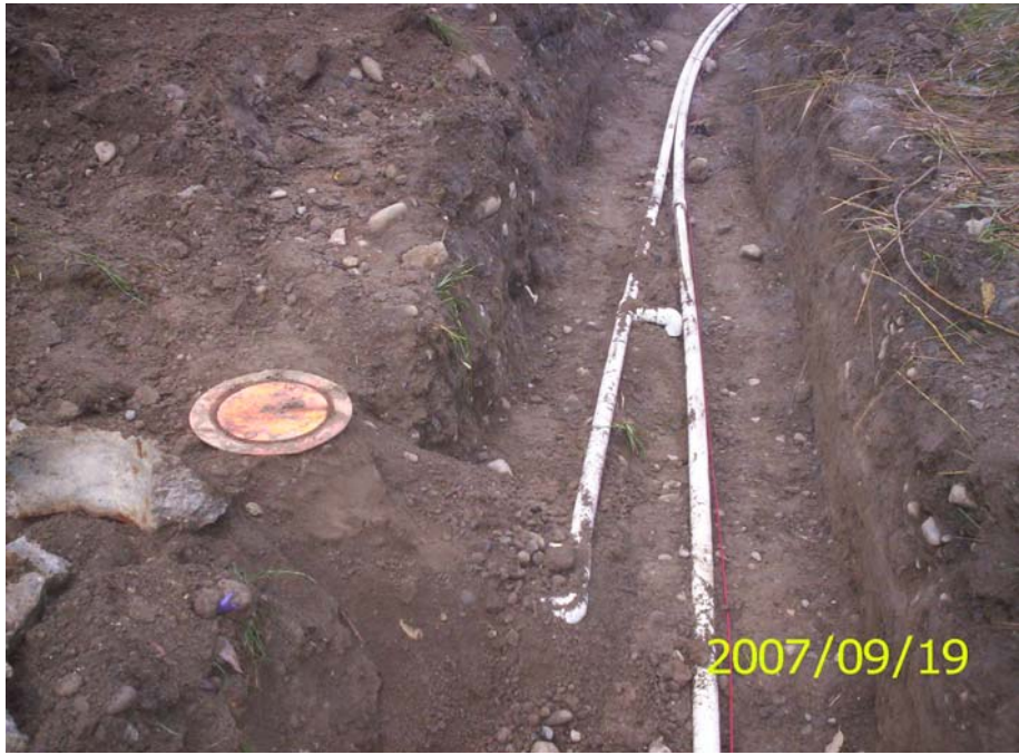
Photo 10: PVC conduit for VWP cables at BH3A/B, near PW1, looking west.
