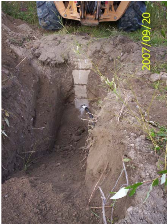
Photo 20: Pump discharge line at manhole barrel and sewer drain at PW4.
