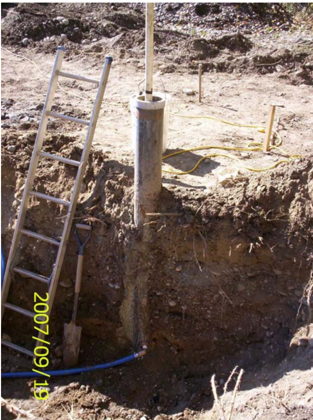
Photo 18: PW5 with pitless adapter and discharge line.
