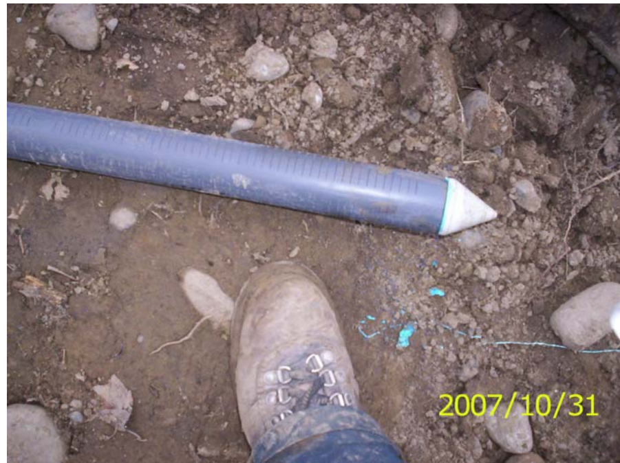
Photo 29: PVC horizontal drain pipe with end cap prior to install.
