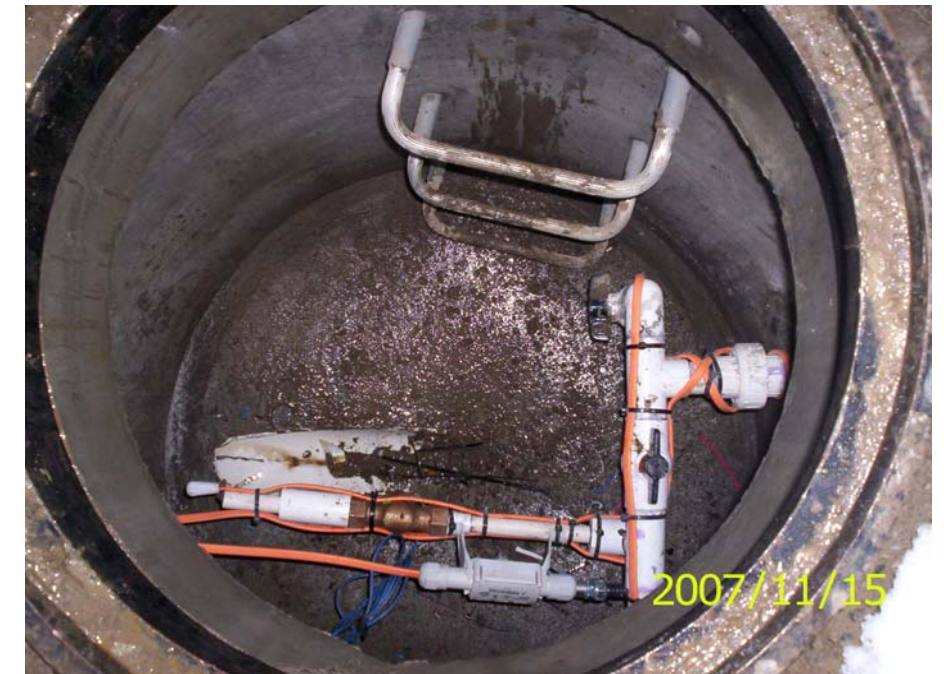
Photo 33: Discharge at HD4 with inline flow meter and heat tape.
