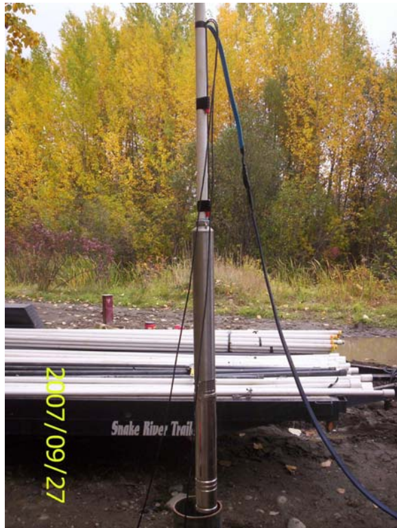
Photo 21: Pump prepared for installation at PW5 with power, ground, and shut-off cables visible.
