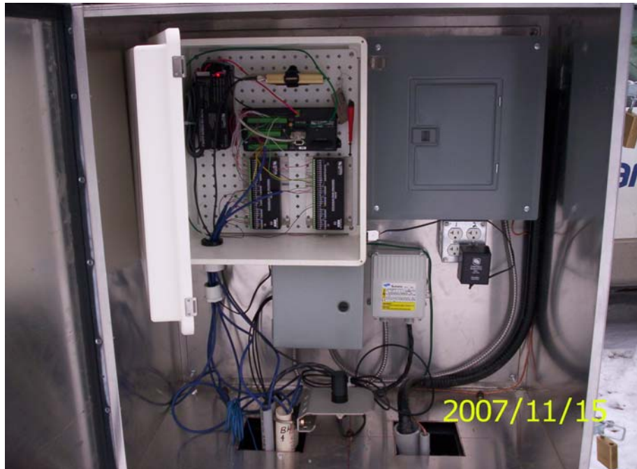
Photo 24: Complete datalogger housing with datalogger, pump controls, breaker panel, cellular antenna visible.
