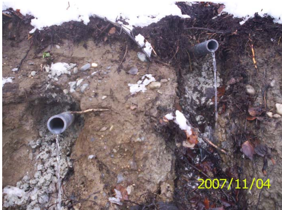
Photo 31: Horizontal drains at HD4 upon completion of drilling.
