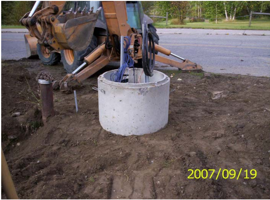
Photo 12: VWP cables and electrical conduit installed at PW1.
