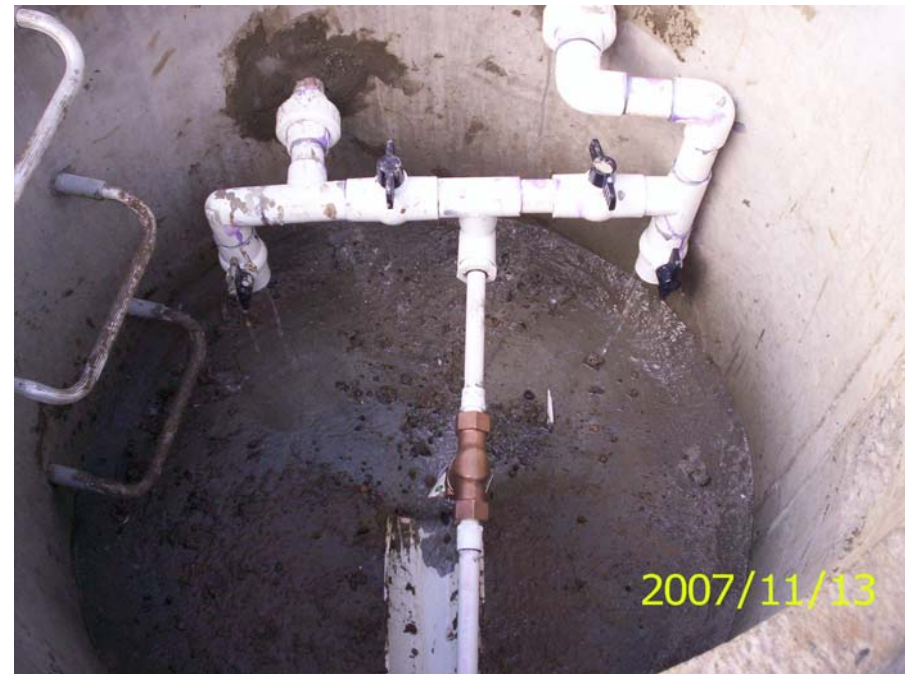
Photo 32: Horizontal drains at HD4 discharge.
