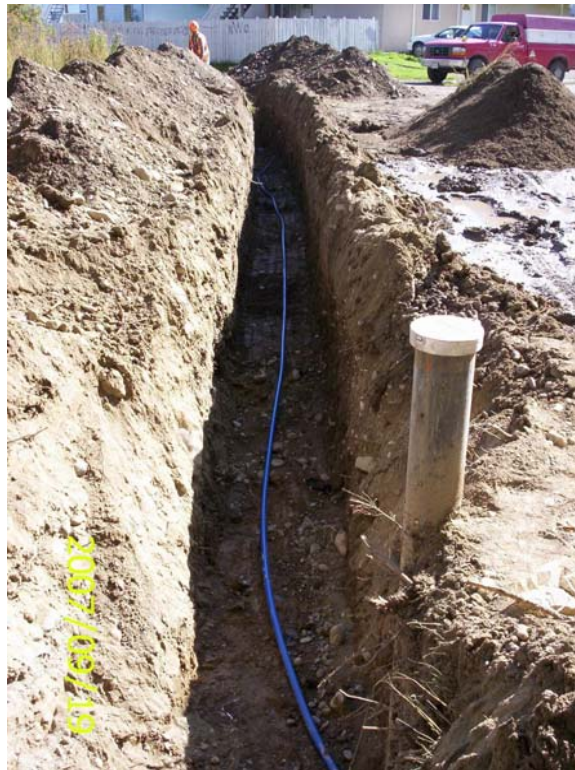
Photo 19: Pump discharge line at PW5.
