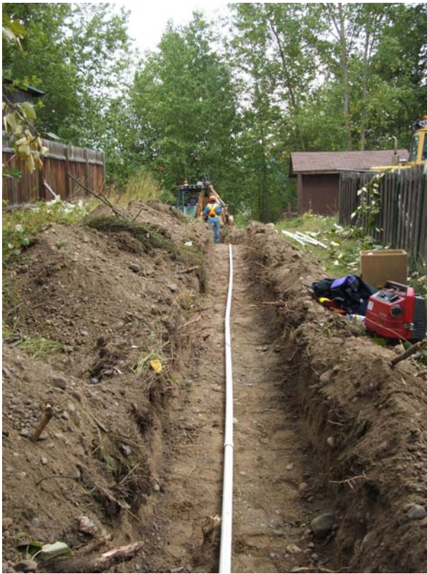
Photo 14: Trenching and VWP conduit installation near BH23.
