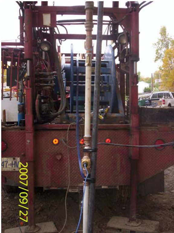
Photo 22: Pump installation at PW5 with flow meter and restrictor visible.
