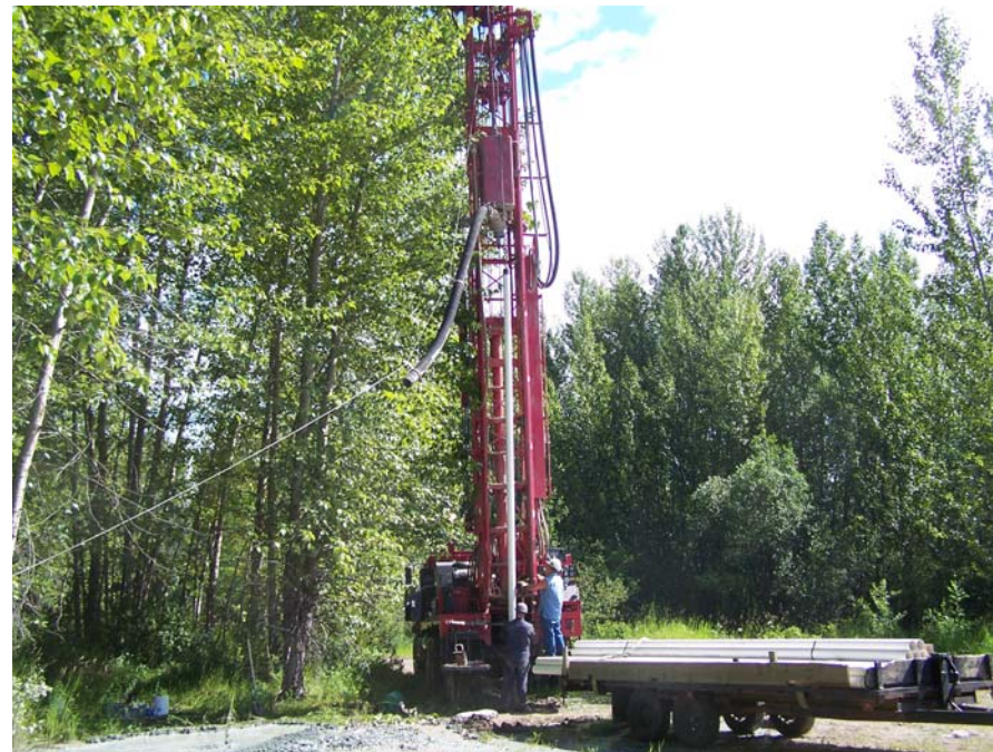
Photo 5: Installing well casing at PW5.
