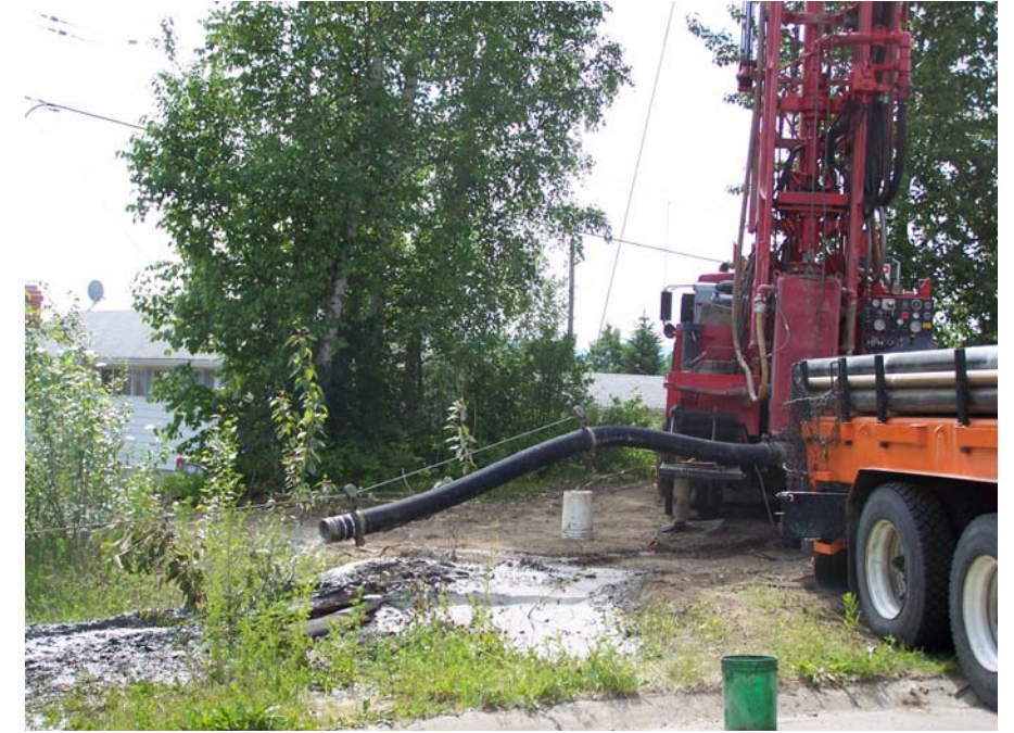
Photo 3: Pumping well development at PW4.
