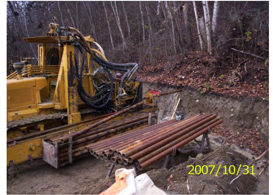
Photo 27: Horizontal drilling at HD4.
