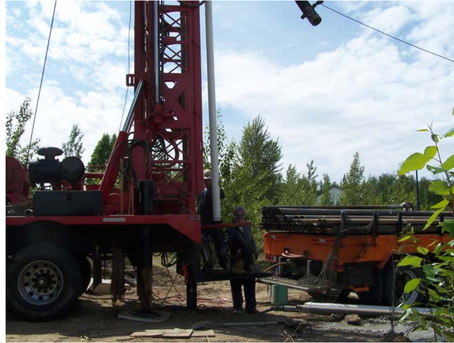
Photo 2: Installing well screen at PW4.
