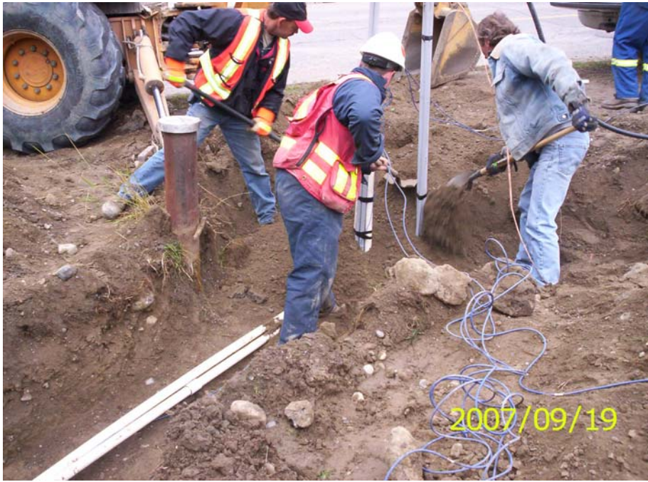
Photo 11: Installing conduit for VWP cables and electricity at PW1.
