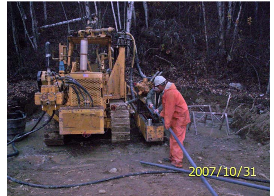
Photo 30: Installing PVC drain at HD4.
