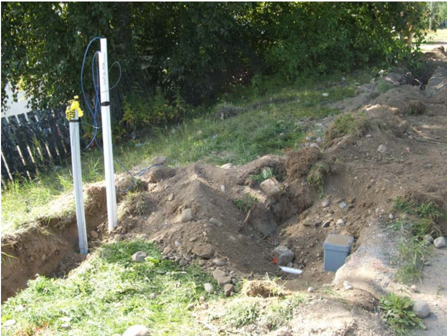
Photo 15: Vibrating wire piezometer installation at BH21
