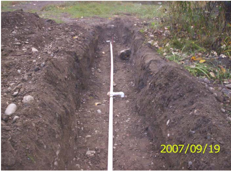
Photo 9: PVC conduit running from BH4B/C near PW1.
