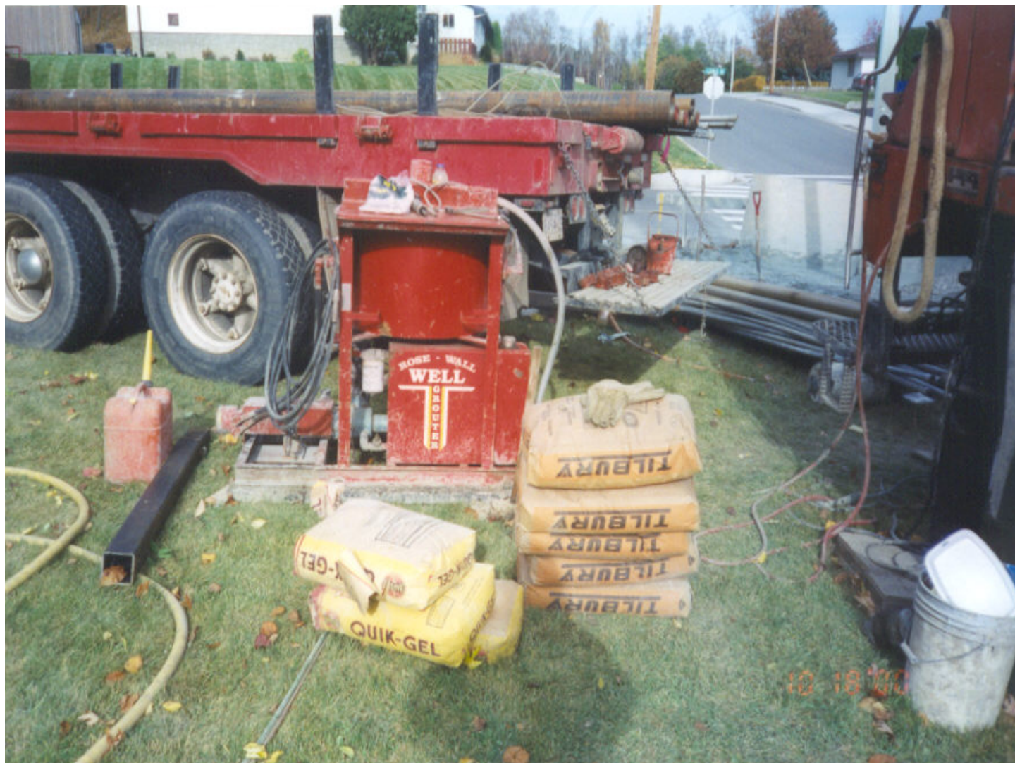
Photo 5: Grout Mixer and supplies taken at SI-7 located at Lewis Drive and Pierce Crescent
