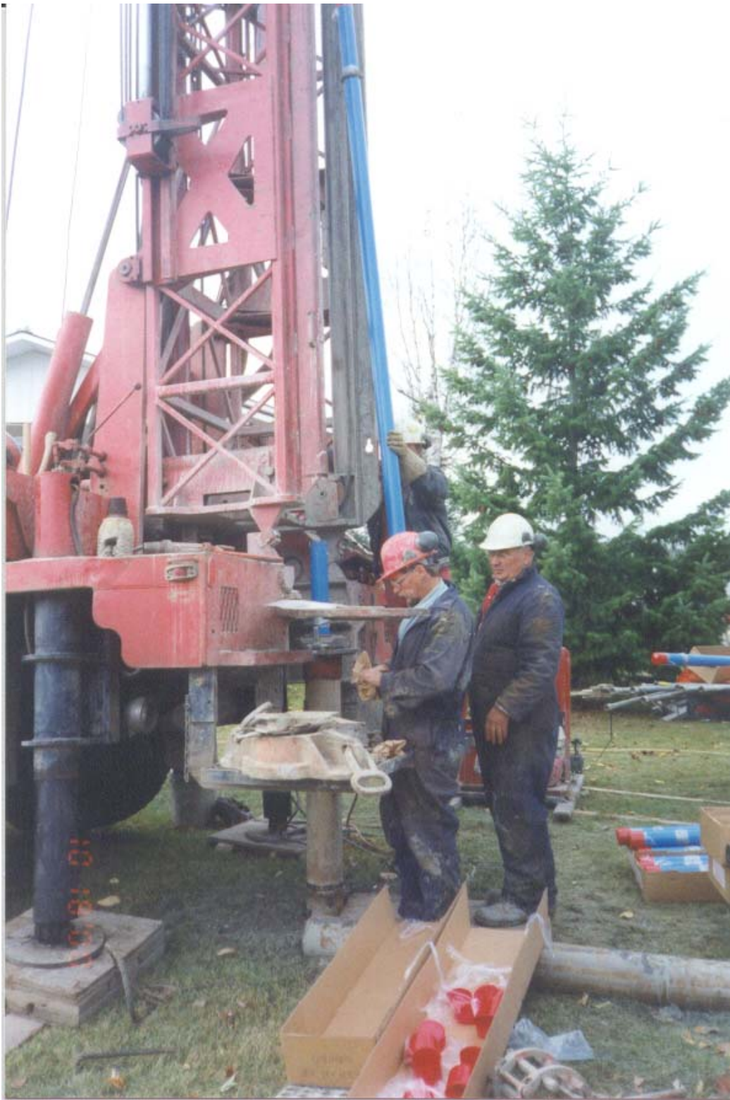
Photo 4: Installing SI Pipe in SI-7 at Lewis Drive and Pierce Crescent
