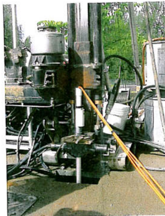
Photo 2: View of vibrating wire piezometer prior to installation in borehole.
