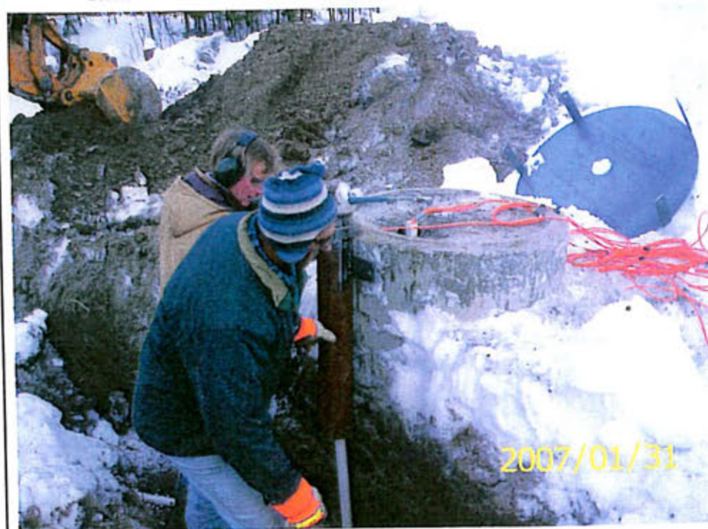
Photo 4: Re-routing of vibrating wire piezometer cable during datalogger installation at BH16.
