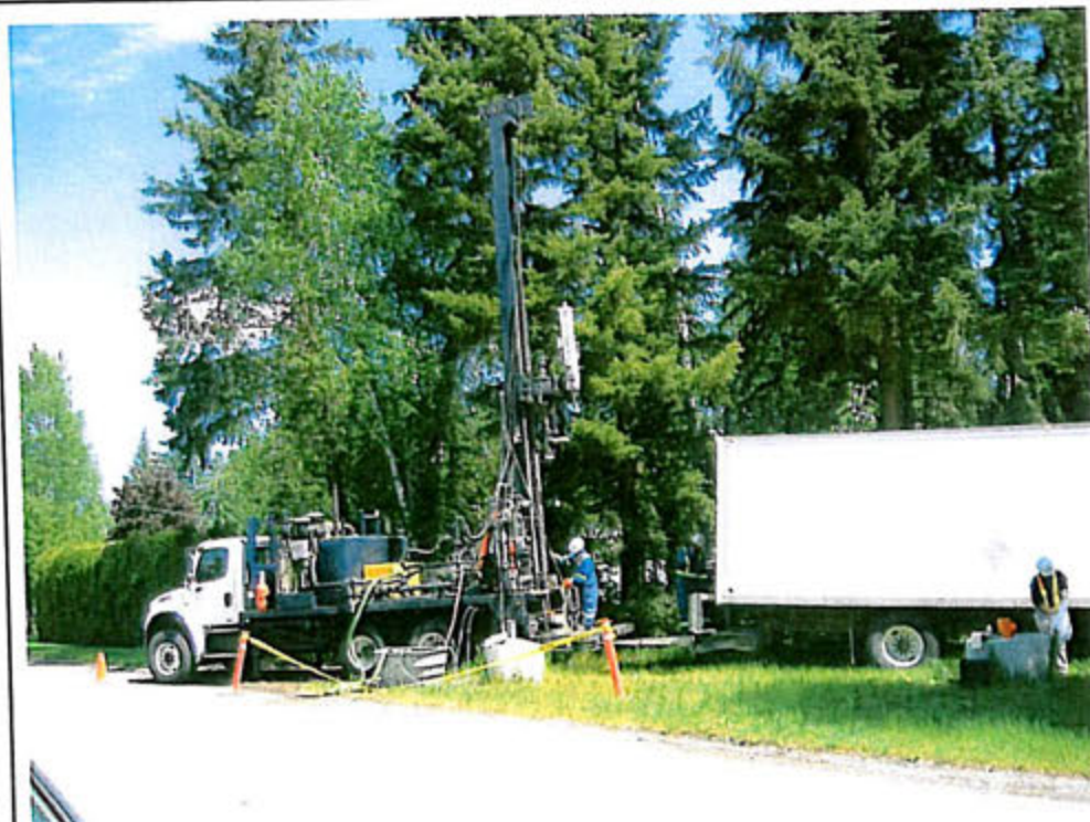
Photo 1: Drilling borehole for installation of vibrating wire piezometer 8A.
