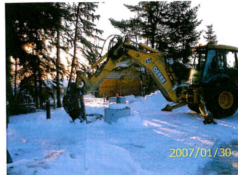
Photo 3: Trenching between vibrating wire piezometer locations prior to installation of datalogger system at BH8.
