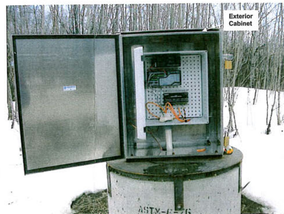
Photo 6: Completed installation of vibrating wire piezometer and datalogger system at BH16.
