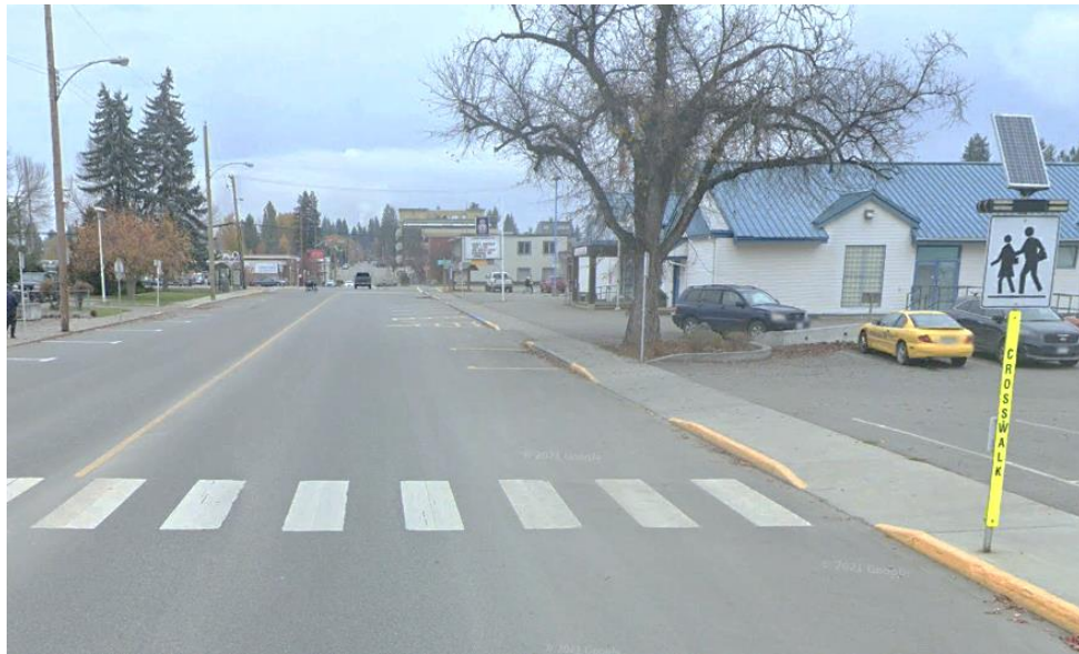
Figure 19: Existing Crosswalk with RRFBs, Kinchant Street
