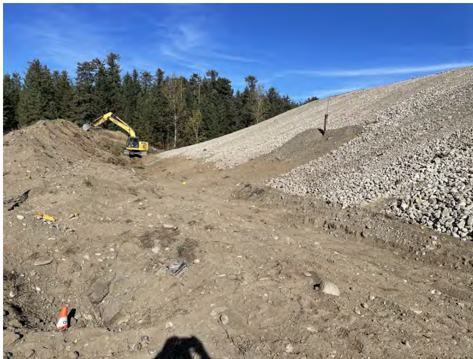
PHOTOGRAPH 5: Looking north. OW-6 after new toe berm (18 October 2022)
