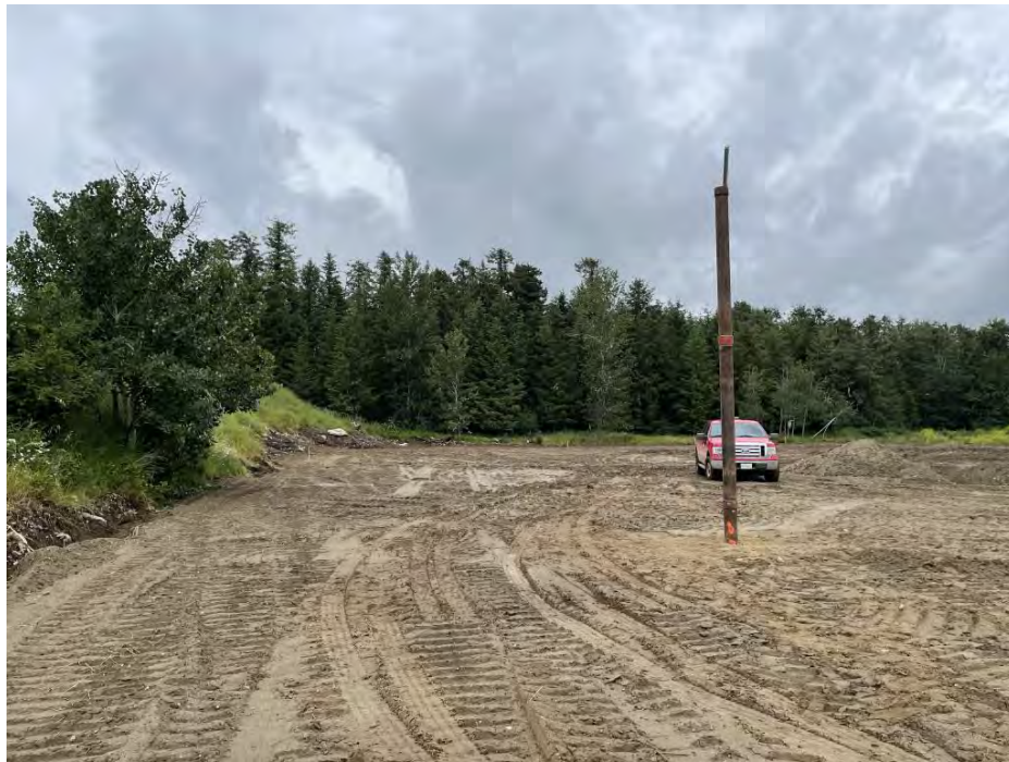
PHOTOGRAPH 4: Looking north. OW-6 extended to accommodate new toe berm.
