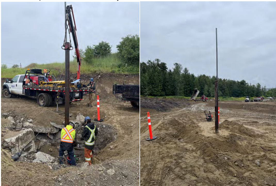
PHOTOGRAPH 2&3: Upgrading OW-6 by extending to new elevation of 537.98 m ASL (30 June 2022).
