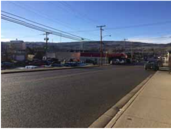
Photo 170: View of crosswalk at St. Laurent and Vaughan – does not line up with curb ramp and cracked pavement (view from NE corner looking south)
