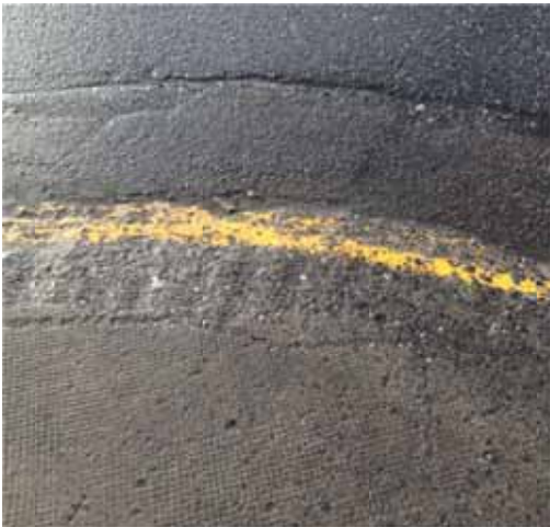
Photo 230: Crosswalk – looking south (from NW corner by Safeway) – rough/broken pavement and lacks tactile warnings
