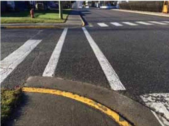
Photo 196: Looking westward at the SE corner of St. Laurent and Wilson – lip/dip at transition
