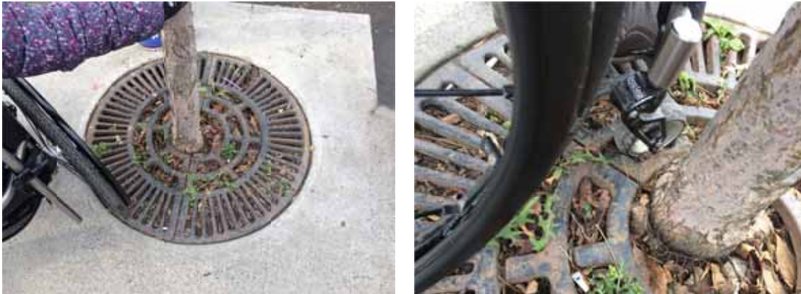
Photo 58: Tree grate openings are too large and are a hazard for mobility devices
