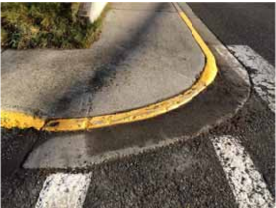
Photo 169: St. Laurent and Vaughan Street (curb ramps at NE corner) – Challenging dips/lips at transition between curb and street
