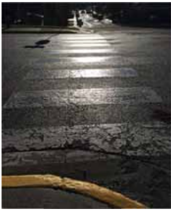
Photo 170: View of crosswalk at St. Laurent and Vaughan – does not line up with curb ramp and cracked pavement (view from NE corner looking south)
