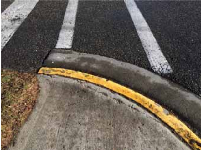
Photo 193: Steep curbs on the NE corner
