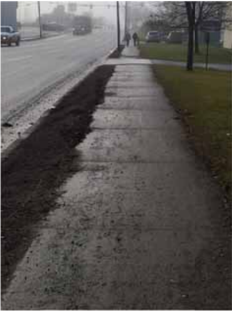
Photo 226: Heading south (on the western side of the street) there is a broken sidewalk that narrows the pathway – still about 14220 mm wide, more broken sidewalks
