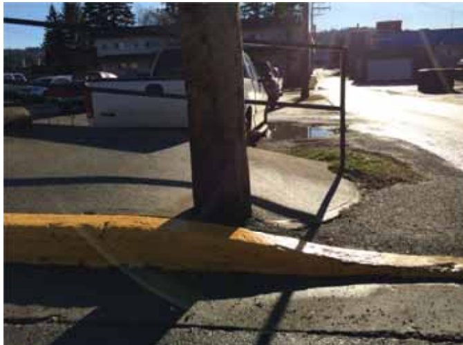
Photo 162: Curb ramp on south side very steep -- Alison had to back down it & pole narrows pathway
