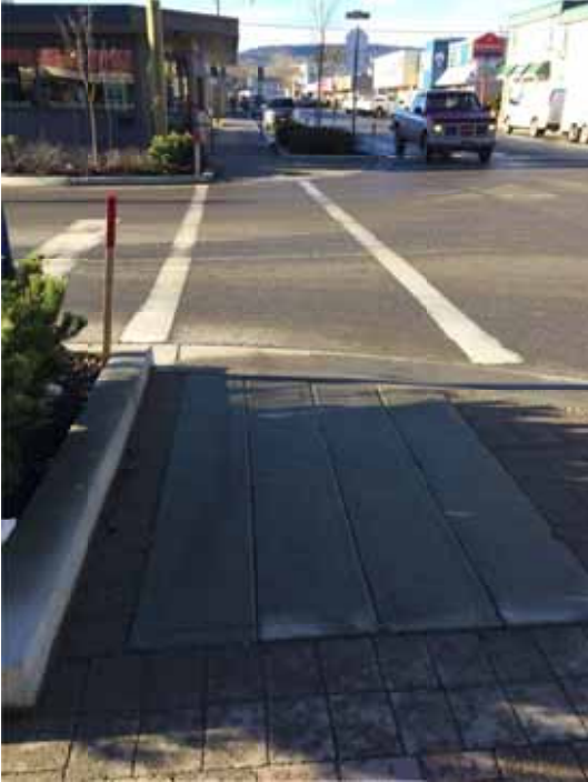
Photo 157: Kinchant Street and St. Laurent (curb on the SW corner with tactile lines)
