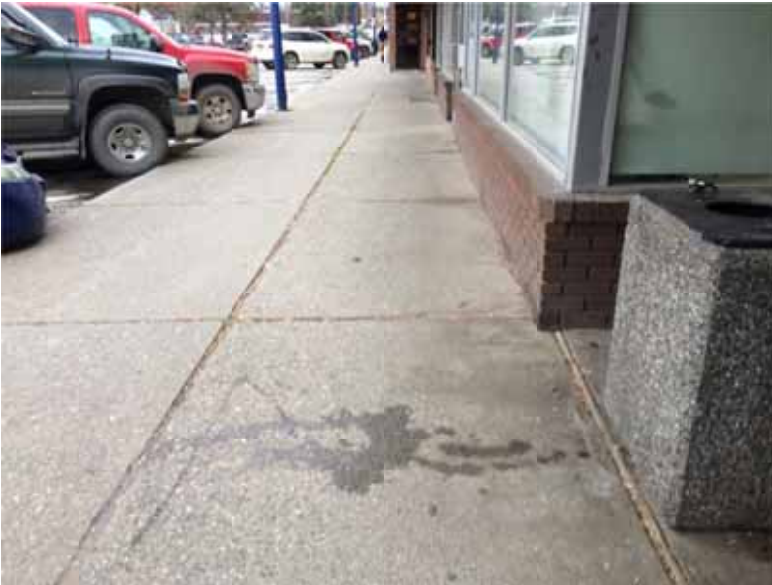
Photo 23: Spacious walkway on Reid Street that is approximately 1.8 m wide where street furniture (e.g. garbage bin) is kept outside the accessible path of travel
