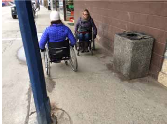
Photo 103: Combination of garbage bin and pole narrow path of travel
