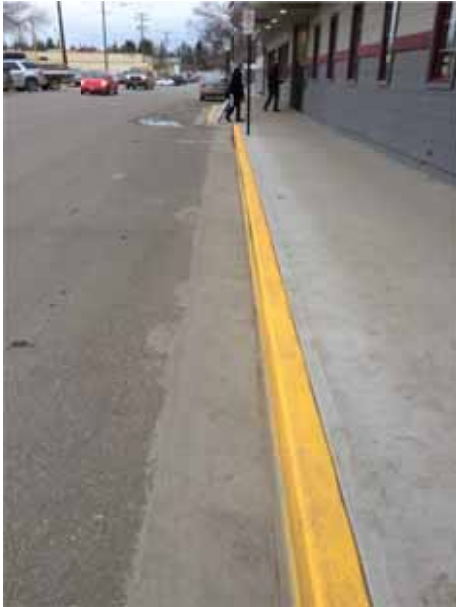
Photo 220: SE corner – Dip/Lip in transition & no tactile warnings
