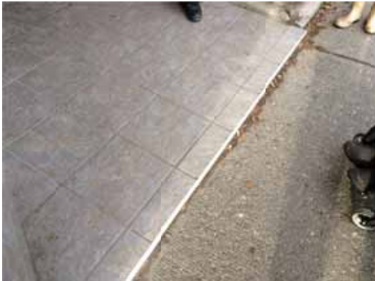
Photo 86: Ramp leading up to Granville's Coffee has a lip
