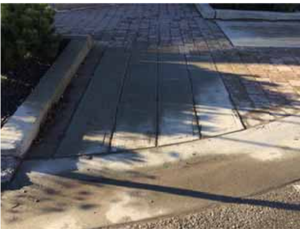
Photo 157: Kinchant Street and St. Laurent (curb on the SW corner with tactile lines)
