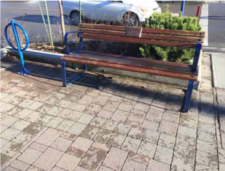
Photo 149: Heading east on north side sidewalk of St. Laurent towards the Ramada – new sidewalk with abrupt transitions in between concrete sections
