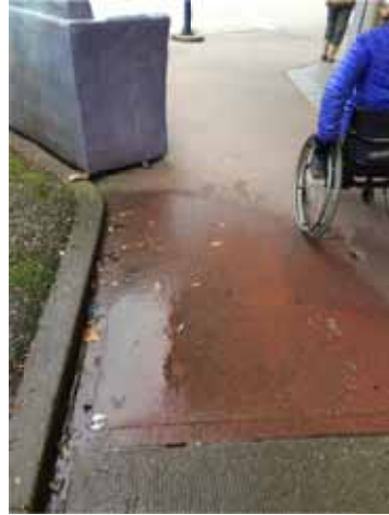
Photo 32: Puddle forming by Willis Harper may become an ice hazard
