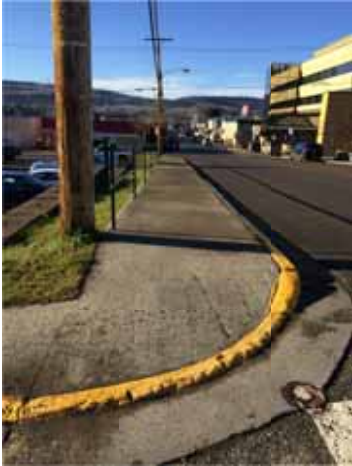
Photos 174: St. Laurent Ave and Vaughan St (on the SW corner) – Cracked concrete and steep lip/dips
