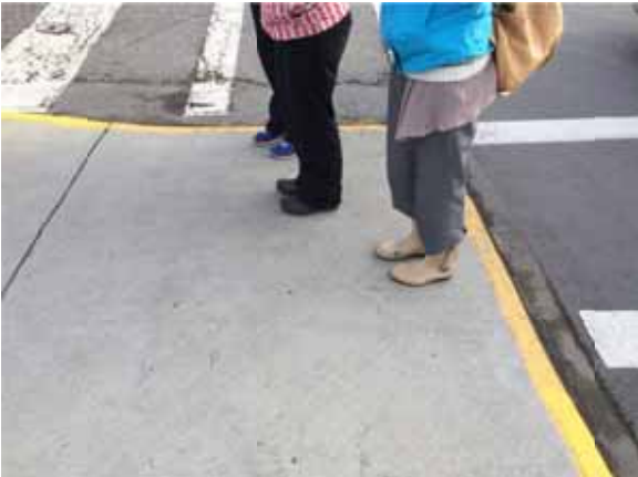
Photo 42: NW corner of Shepherd Ave and Reid St – Lip/gap at transition between roadway and curb ramp
