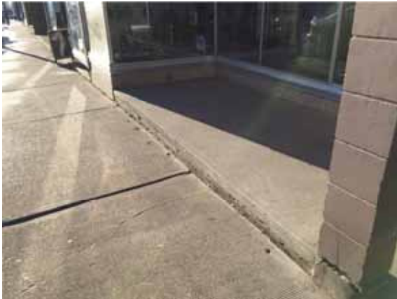
Photo 105: Abrupt transition by Keen's Sports -- could use yellow paint to improve visibility
