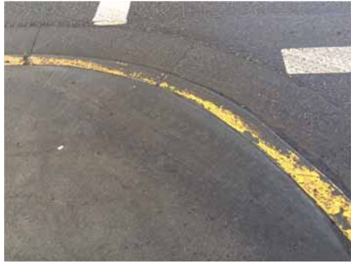
Photo 224: Southeast corner has a better curb ramp and push button but lacks tactile indicators for people with low vision
