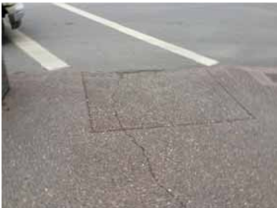
Photo 96: NE corner of Reid St and Barlow Ave looking south - Curb ramp with cracked concrete
