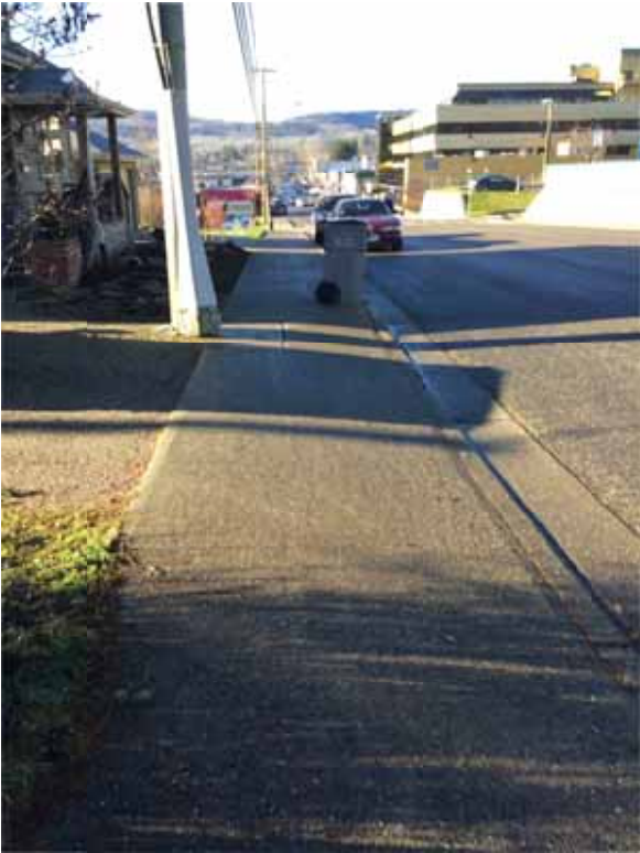
Photo 179: Challenging cross slopes heading downhill on south side
