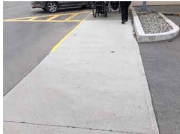
Photo 111: New section of concrete by Chevron Station
