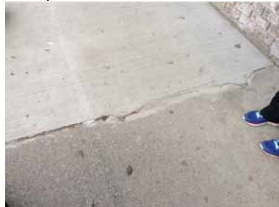
Photo 53: Cracked pavement in front of Subway
