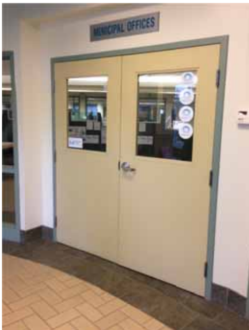
Photo 14: Interior entrance doors
