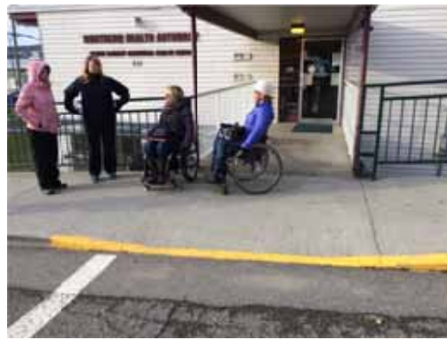
Photo 26: Curb ramp by Health Unit on Reid Street provides access between the street and sidewalk for people using mobility devices, but may be difficult to detect for someone with low vision and narrows the clear path of travel
