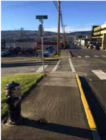
Photo 172: SE Curb has significant incline and dips/lips at the transition point
