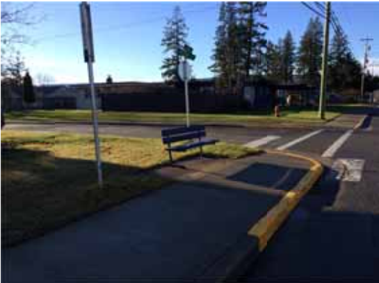
Photo 196: Looking westward at the SE corner of St. Laurent and Wilson – lip/dip at transition
