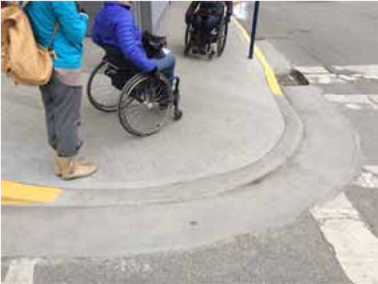
Photo 217: NE corner of Barlow Ave and McLean St by Billy Barker Casino – the pole blocks visibility, there is a lip/dip on the curb ramp, no tactile warnings for people with low vision
