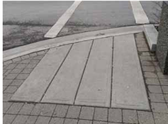
Photo 64: NW corner of Reid St. and St. Laurent Ave looking south with tactile lines
