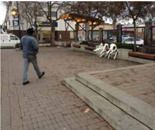
Photo 70: Limited colour contrast and no tactile warnings on Spirit Square steps
