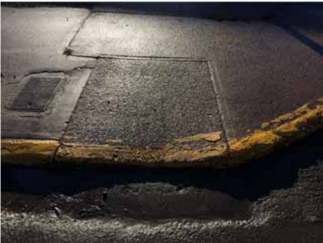
Photo 123: SE corner of Reid St. and Carson Ave -- lacks proper curb ramp
