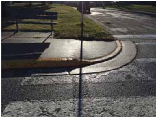
Photo 197: St. Laurent and Wilson Intersection (curb ramps at the SW corner) – lip/dip at transition
