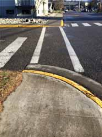
Photo 192: Wilson St and St. Laurent Ave (looking south from NE corner) – Rough concrete
