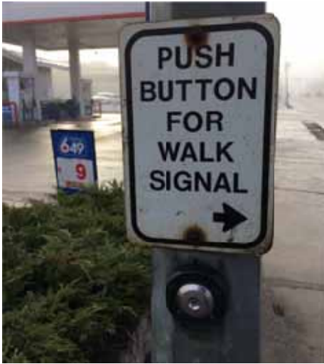
Photo 224: Southeast corner has a better curb ramp and push button but lacks tactile indicators for people with low vision
