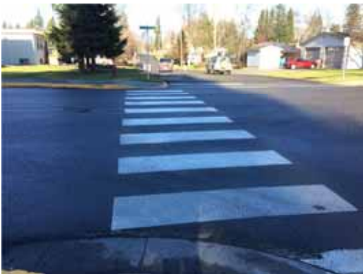
Photo 206: View of crosswalk across St. Laurent from the SW corner – lacks tactile warnings
