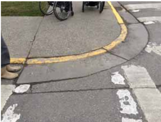
Photo 220: SE corner – Dip/Lip in transition & no tactile warnings
