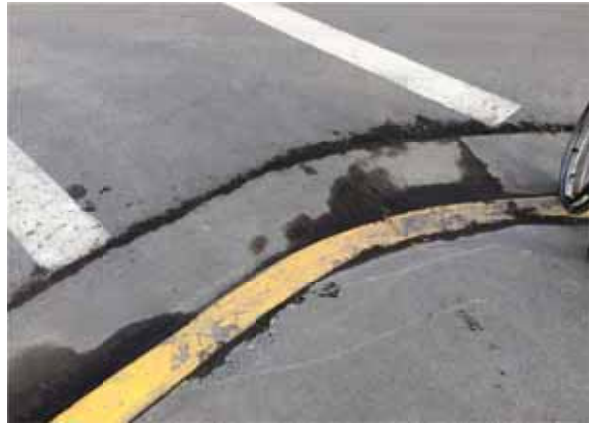
Photo 42: NW corner of Shepherd Ave and Reid St – Lip/gap at transition between roadway and curb ramp
