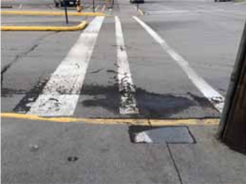
Photo 40: NE corner of Shepherd Ave and Reid St connected to crosswalk leading to SE corner – Manhole, cracked concrete, lip
