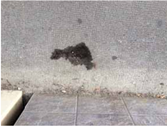
Photo 82: Damaged sidewalk in front of Granville's Coffee
