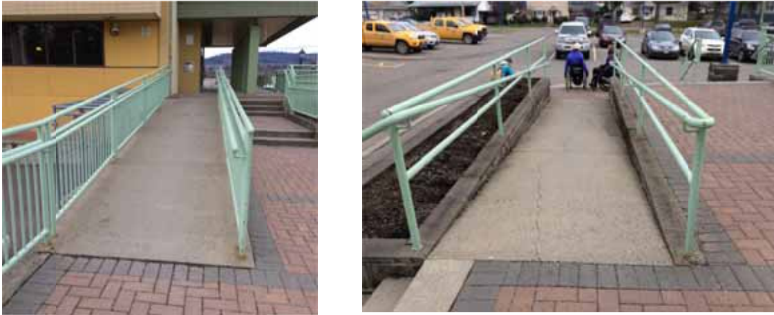
Photo 10: Accessible exterior pathway connecting parking lot to main entrance with ramps
