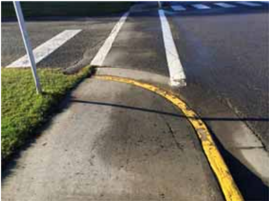
Photo 206: View of crosswalk across St. Laurent from the SW corner – lacks tactile warnings
