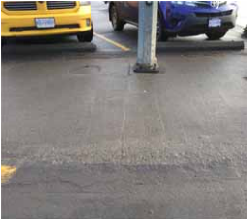
Photo 229: Curb ramp on Safeway side has rough pavement and lacks tactile indicators
