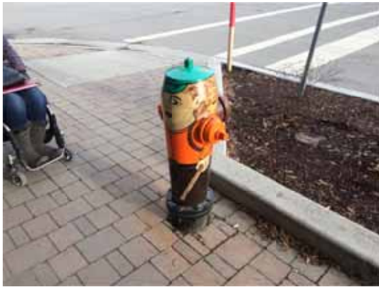
Photo 69: Uneven sidewalk surface and limited colour contrast around planting bed
