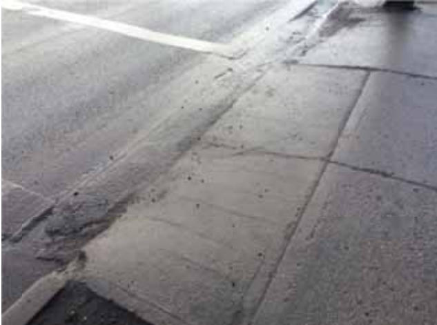
Photos 227: St. Laurent St and Front St northwest corner – Can only cross on the north side; good curb ramp; push button is at located at a good height; lacks tactile warnings for people with low vision
