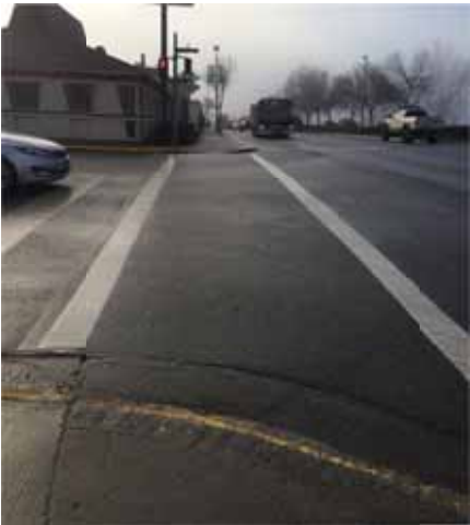
Photo 230: Crosswalk – looking south (from NW corner by Safeway) – rough/broken pavement and lacks tactile warnings
