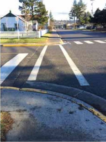
Photo 182: Very steep curb (NE Corner) with no tactile warnings for people with visual disabilities
