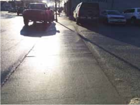
Photo 108: The alley may create a hazard for people with low vision because there is limited tactile and visual warning of it
