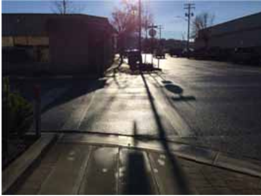
Photo 145: Crosswalk along St. Laurent at McLean Street (looking south towards Edward Jones from NE corner) with tactile lines
