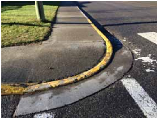
Photo 197: St. Laurent and Wilson Intersection (curb ramps at the SW corner) – lip/dip at transition
