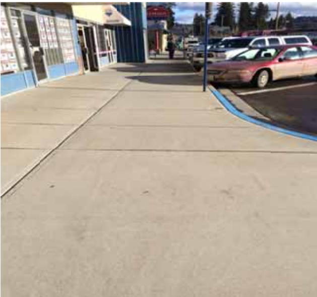
Photo 149: Heading east on north side sidewalk of St. Laurent towards the Ramada – new sidewalk with abrupt transitions in between concrete sections
