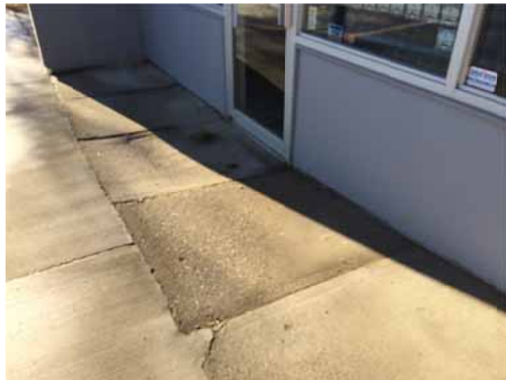
Photo 107: Dip in concrete by Fraser Broughton CPA Office
