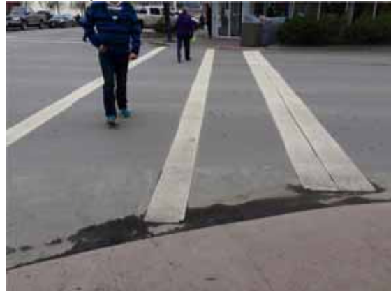
Photo 99: Crosswalk connecting Scotiabank to Willis Harper (Home Hardware)
