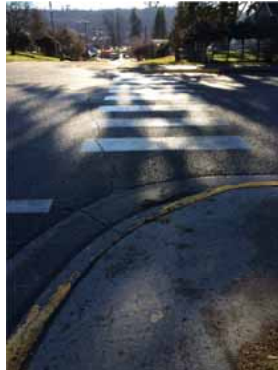
Photo 183: St. Laurent and Callanan Street – Looking south from the NE corner at cross walk going across St. Laurent – rough/broken concrete
