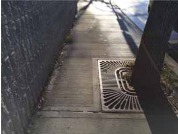
Photo 24 Tree grate narrows the accessible path of travel on McLean St sidewalk (by St. Laurent Ave). The gaps in the tree grate are also too large and hazardous for people using mobility devices
