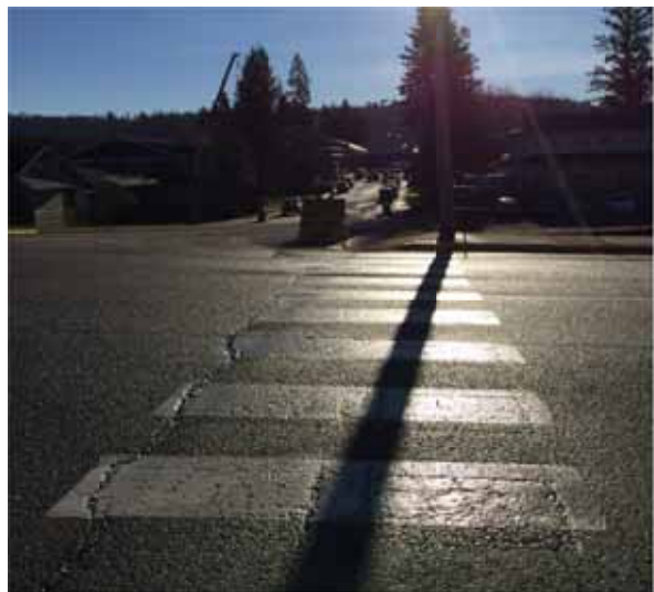
Photo 166: Crosswalk at Vaughan and St. Laurent (looking south) does not line up with curb ramp
