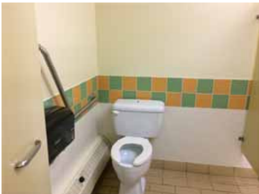
Photo 22: Accessible stall in men's washroom may not have enough space for someone using a larger mobility device such as a scooter or larger power wheelchair
