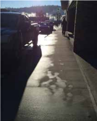
Photo 102: New sections of concrete sidewalk (Bell Store to Integris Credit Union)
