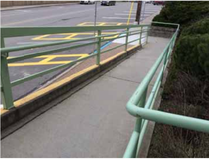
Photo 11: Designated accessible parking stalls on Kinchant St.
