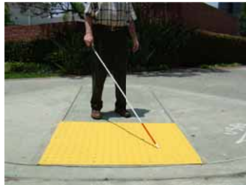
Photo 29: Example using detectable warnings/tactile walking surface indicators/truncated domes to warn people with visual disabilities about the presence of a curb ramp
