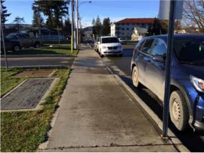
Photo 209: Heading westward on St. Laurent Ave. away from Dunrovin Park Lodge on the south side – unmarked driveways and curb ramps
