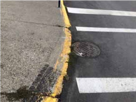
Photo 40: NE corner of Shepherd Ave and Reid St connected to crosswalk leading to SE corner – Manhole, cracked concrete, lip
