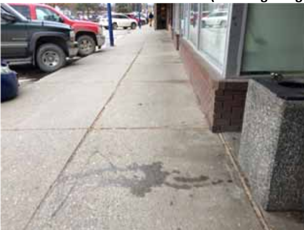
Photo 47: Wide spacious path of travel with ample space for two mobility devices to pass by each other where street furniture (i.e. the garbage bin) is kept outside the accessible path
