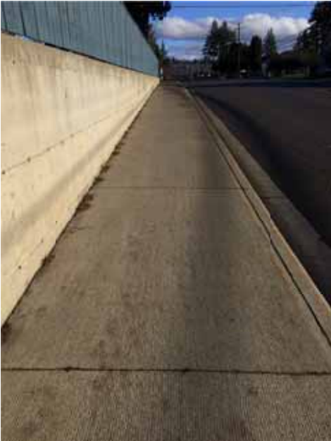
Photo 175: Heading up the steep hill eastward on north side
