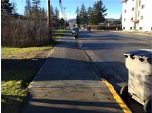
Photo 200: Very bad cross slope between Wilson St and James St
