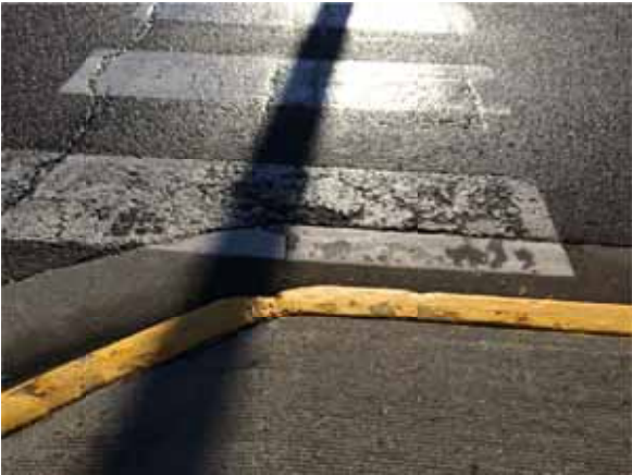
Photo 169: St. Laurent and Vaughan Street (curb ramps at NE corner) – Challenging dips/lips at transition between curb and street
