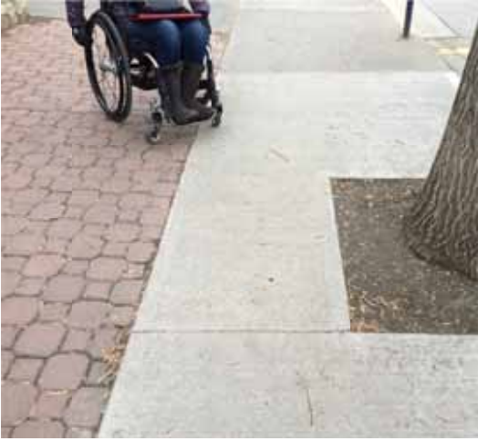
Photo 214: Looking eastward towards the provincial office – tree grates are inaccessible
