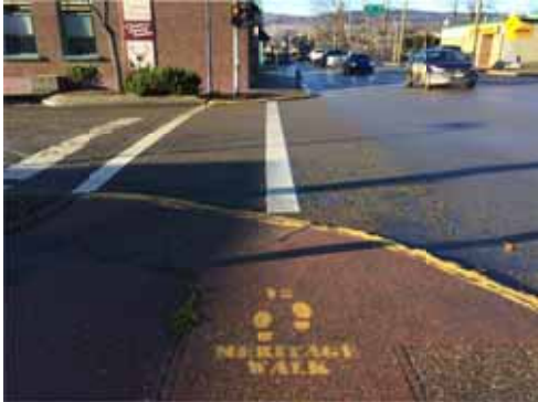
Photo 125: SE corner of Reid St and Carson Ave (facing west) has heritage walk foot prints
