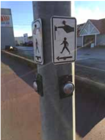
Photo 124: Pedestrian push buttons on SE corner
