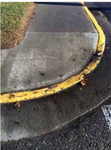
Photo 182: Very steep curb (NE Corner) with no tactile warnings for people with visual disabilities
