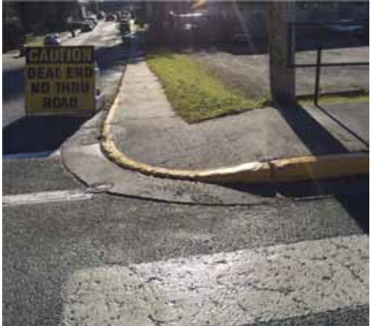
Photos 174: St. Laurent Ave and Vaughan St (on the SW corner) – Cracked concrete and steep lip/dips
