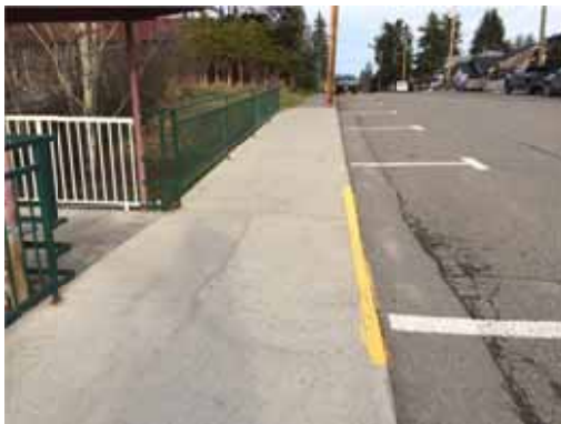
Photo 26: Curb ramp by Health Unit on Reid Street provides access between the street and sidewalk for people using mobility devices, but may be difficult to detect for someone with low vision and narrows the clear path of travel
