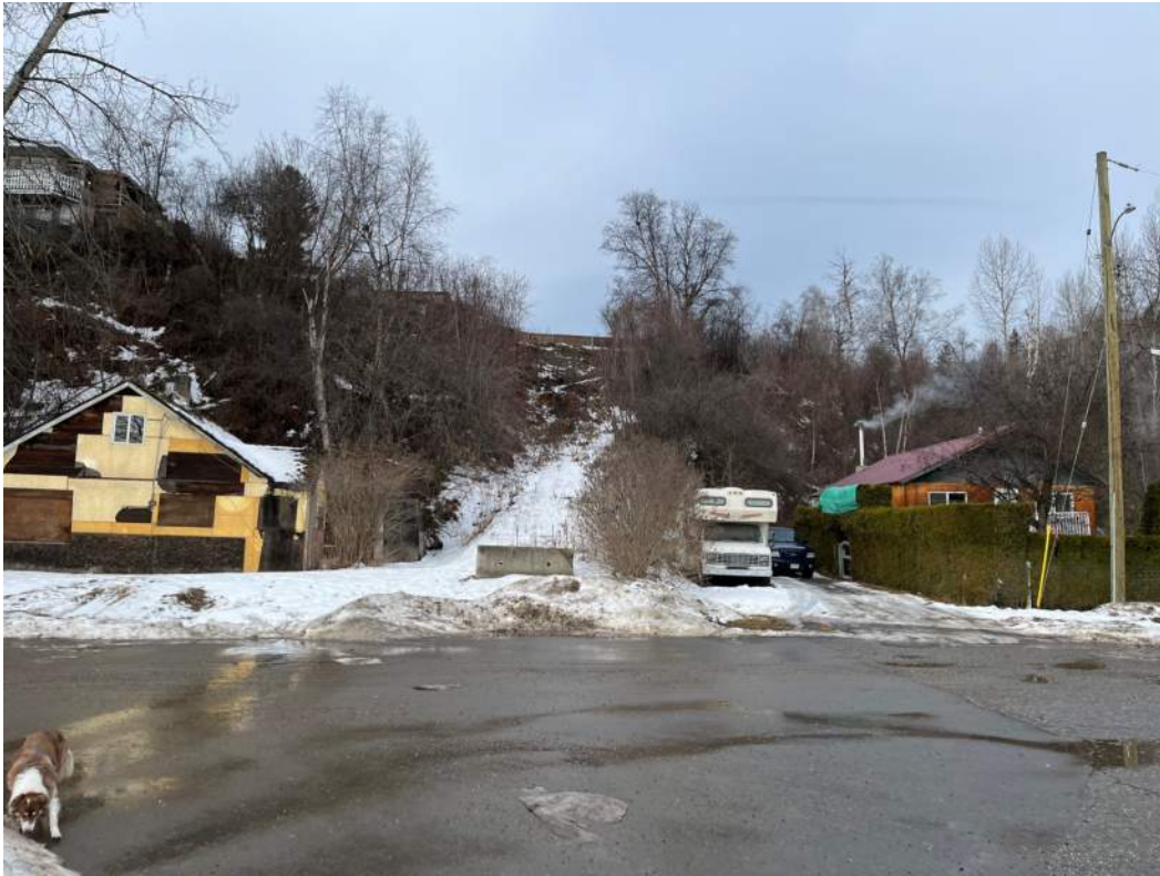
Photo 2: Steep Bank Between the Park and Foster Avenue (looking west).
