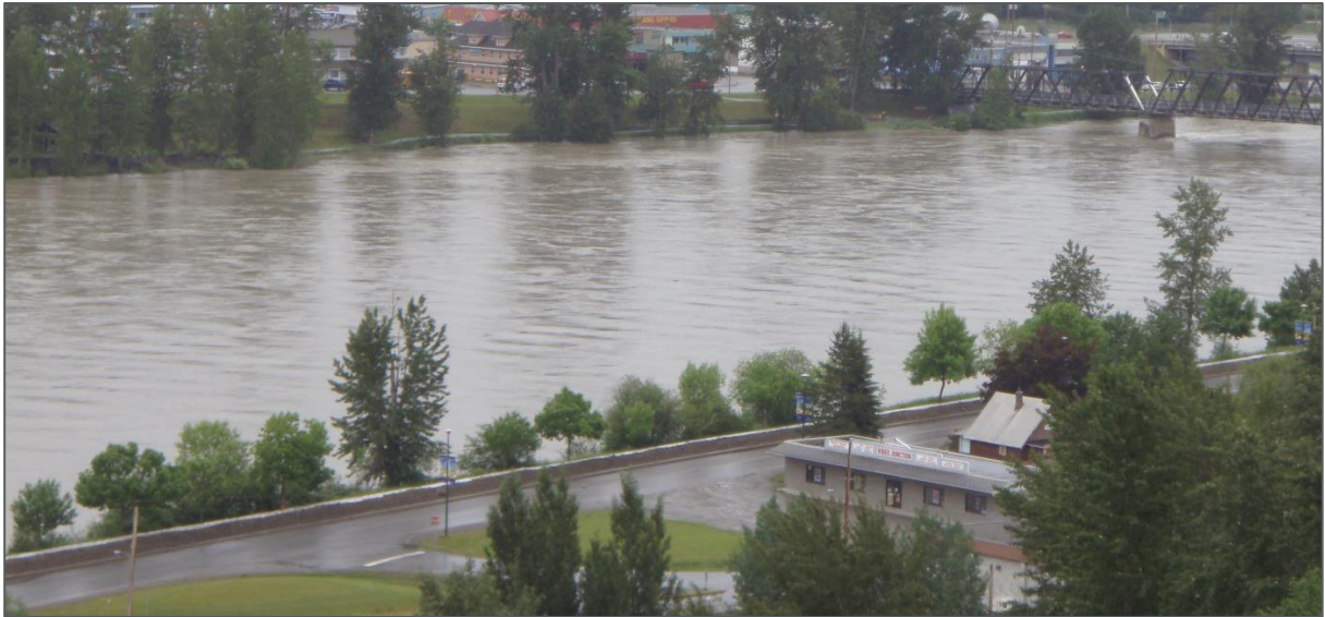
Photo 5 - 2007 – Temporary Flood Protection Along Fraser River Upstream of Bridge Crossings (Source: Urban Systems Ltd.)
