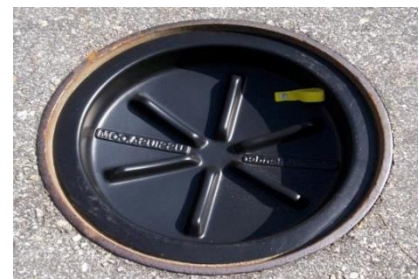
Example Manhole Disk Before Manhole Lid is Installed Photo Source: Manhole Rehab Inc. Website
