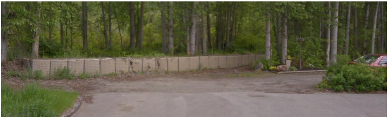
HESCO Barrier Used Along Dragon Creek in 2012 to Protect Against High Creek Water Levels Source: Google Streetview
