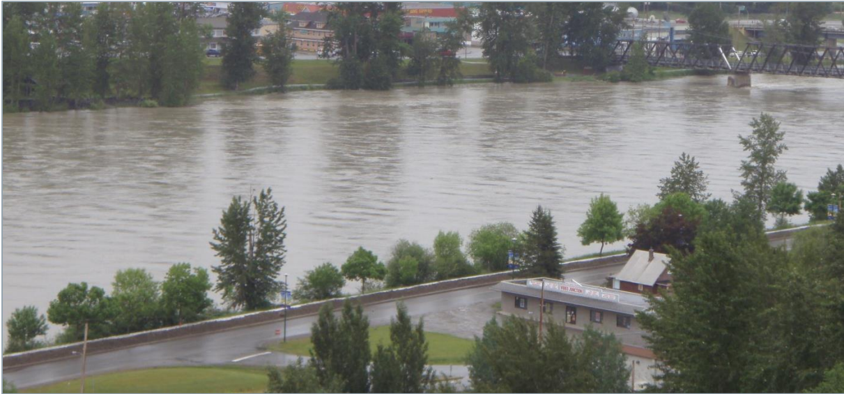
Photo 5 - 2007 – Temporary Flood Protection Along Fraser River Upstream of Bridge Crossings (Source: Urban Systems Ltd.)
