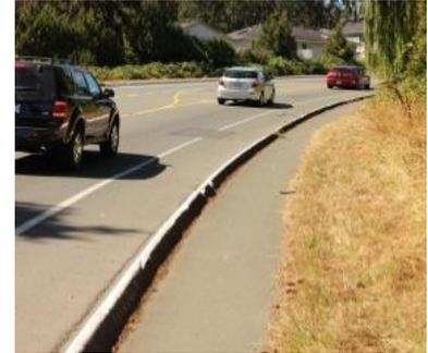
In locations where additional separation may be required, a low-cost option is to install a curb barriers between the shoulder and roadway, these are used in some municipalities in BC as seen in the photo above.
