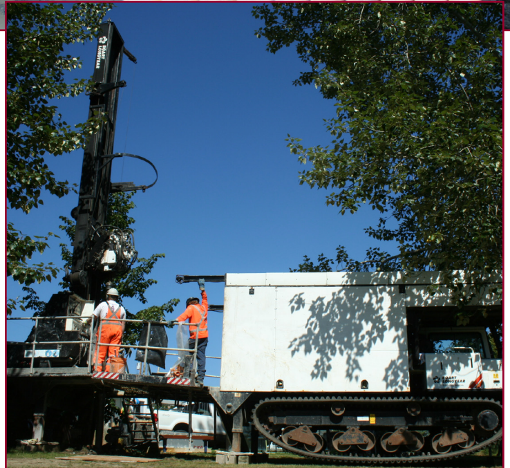
Above, horizontal drilling crews install a series of drains into a hillside off Lewis Drive in West Quesnel. The drains stretch 125 metres or more into the hill, allowing groundwater to flow out of the land stability study area. Right, a series of monitoring wells were installed in 2012 designed to measure the effects of the full-scale dewatering program in the West Quesnel Land Stability study area.
