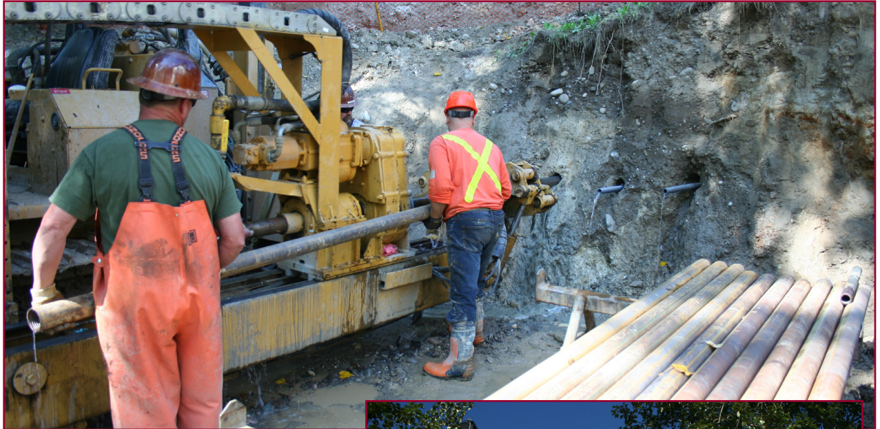
Above, horizontal drilling crews install a series of drains into a hillside off Lewis Drive in West Quesnel. The drains stretch 125 metres or more into the hill, allowing groundwater to flow out of the land stability study area. Right, a series of monitoring wells were installed in 2012 designed to measure the effects of the full-scale dewatering program in the West Quesnel Land Stability study area.
