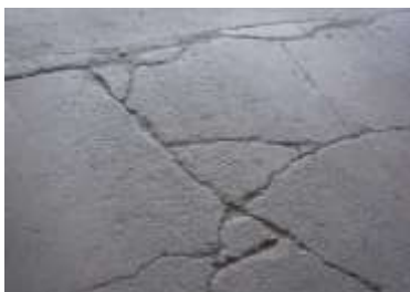
Figure 32 Slab Cracking
