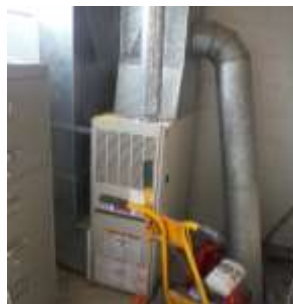
Figure 23 exposed furnace
