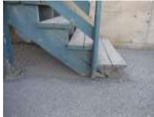
Figure 44 Rear Exit Stair
