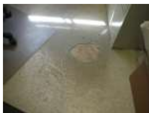
Figure 42 Worn Finishes
