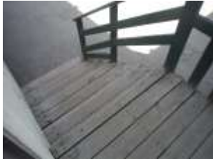
Figure 43 Main Entry Stair
