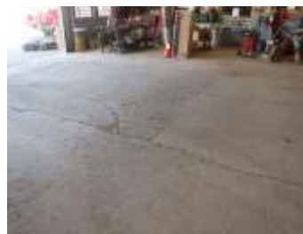
Figure 33 Slab Cracking
