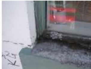
Figure 51 Window Failing
