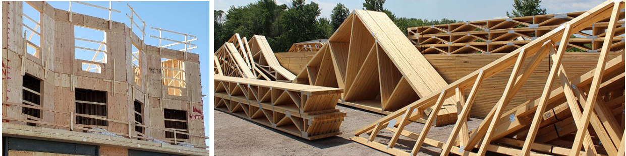
Pre-framed wall panels and trusses (Photos: G. Wimmers, Kingdon Truss)
