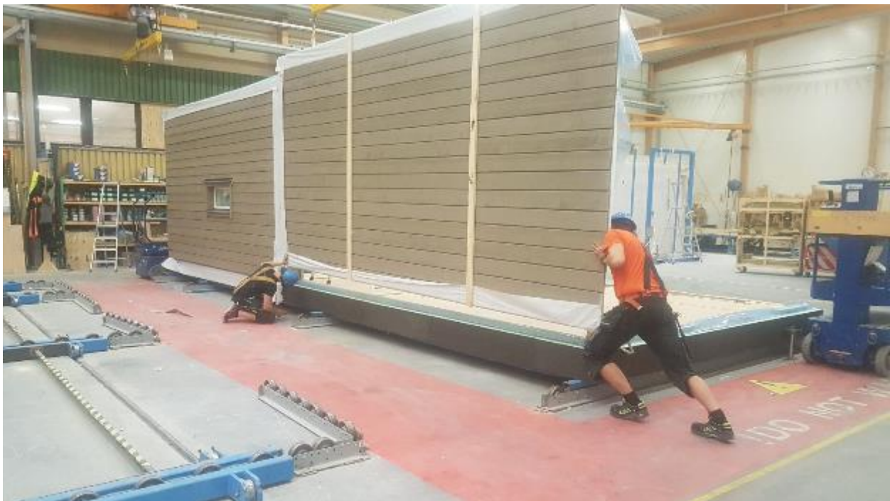
Prefinished walls are mounted on a prefinished floor system during modular construction in Sweden (Photo: G. Wimmers)
