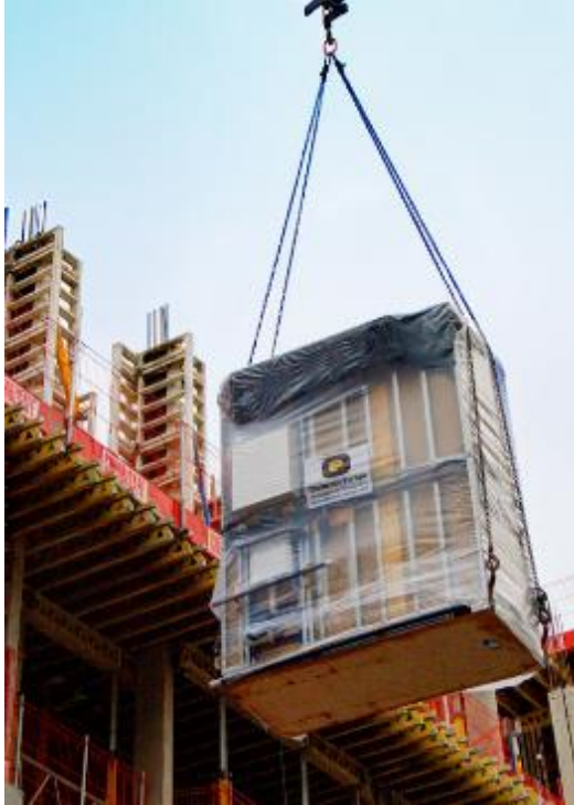
Bathroom Pod lifted into place on building site (Photo: Element Europe)
