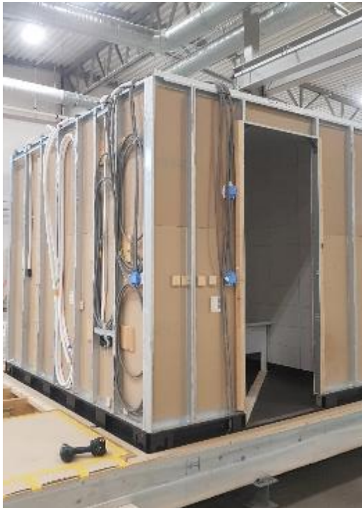
Bathroom pods integrated into module and hooked up to electrical and mechanical services in Sweden (Photos: G. Wimmers)
