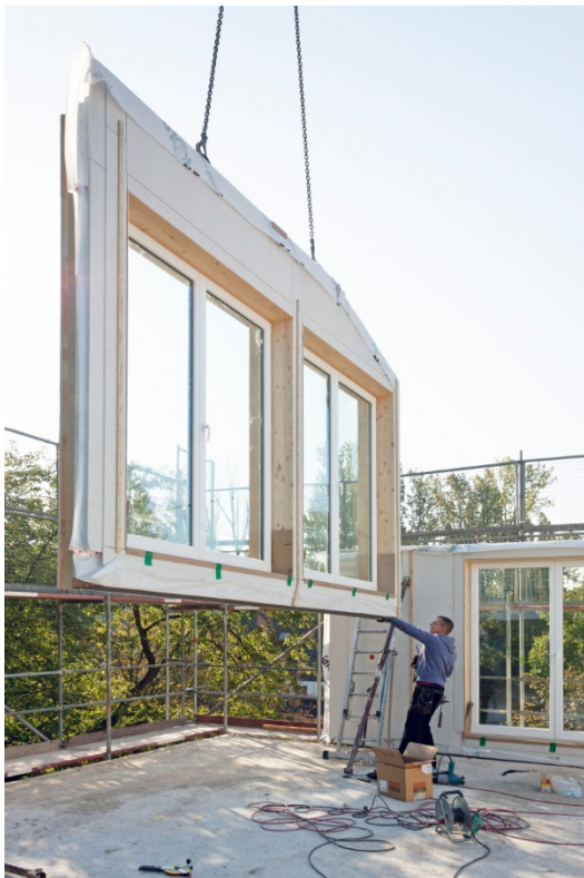
Pre-framed wall panels and trusses (Photos: G. Wimmers, Kingdon Truss)
