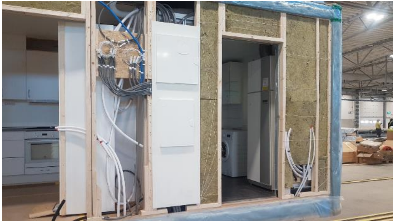
Preinstalled electrical and mechanical systems in module, including the kitchen, heater, warm water and heat recovery ventilation (HRV) in Sweden (Photo: G. Wimmers)
