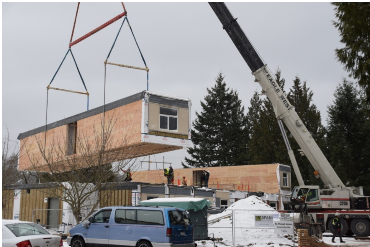
Typical Modular construction in Canada (Photo: Sean Eckford)
