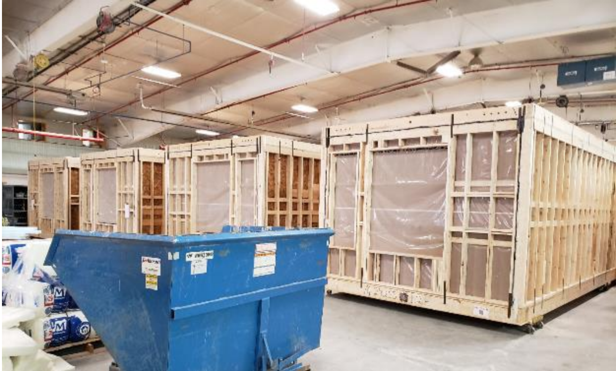
Prefabricated modules featuring completely unfinished walls in Canada (Photo: G. Wimmers)
