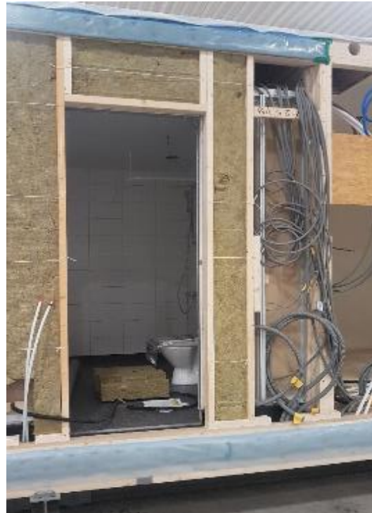
Bathroom pods integrated into module and hooked up to electrical and mechanical services in Sweden (Photos: G. Wimmers)
